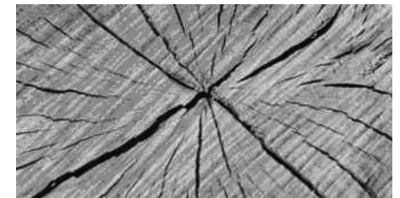
Cracks in wood
