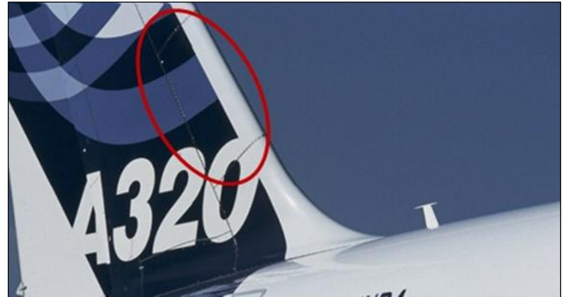
Example of a crack in an aircraft structure
